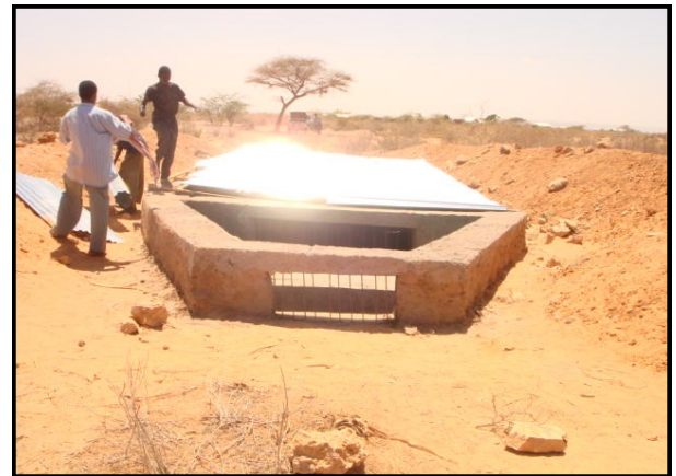
Rehabilitation of a Berkad (water storage tank) in progress In Qabno settlement
