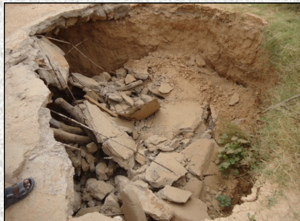
A collapsed water point in Sanaag Region of Somaliland
