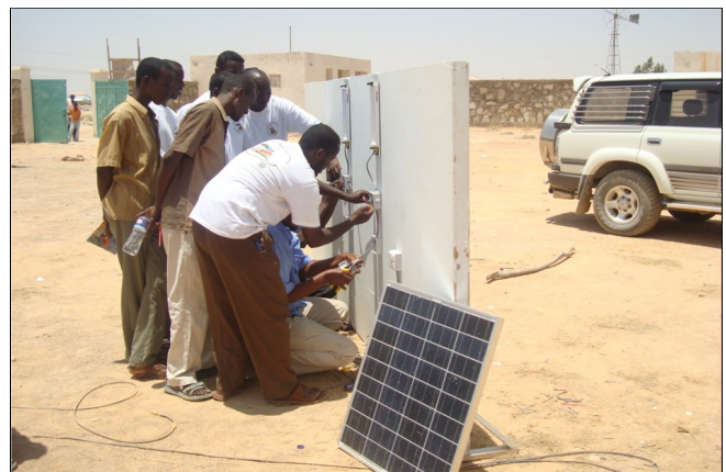
Trainees Learn How to Install a Solar Panel
